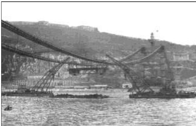
*First roadbed element loaded onto the suspension cables from two barges on the Danube on 14 April 1964.*
