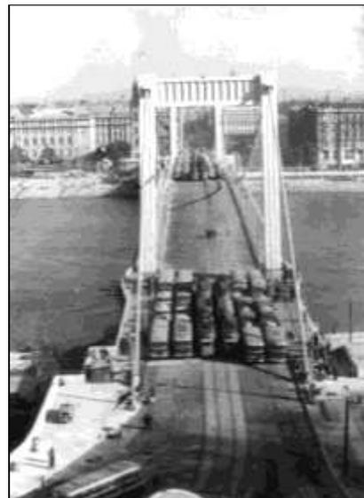
*Second day of the load testing on 16 September 1964. A similar picture of the bridge fully loaded with trams and buses made the wire services and was carried in newspapers across the United States a few days later.*
